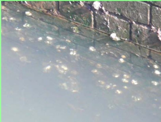
■ Barnacle and Algae were stuck to JR line bridge pier.
