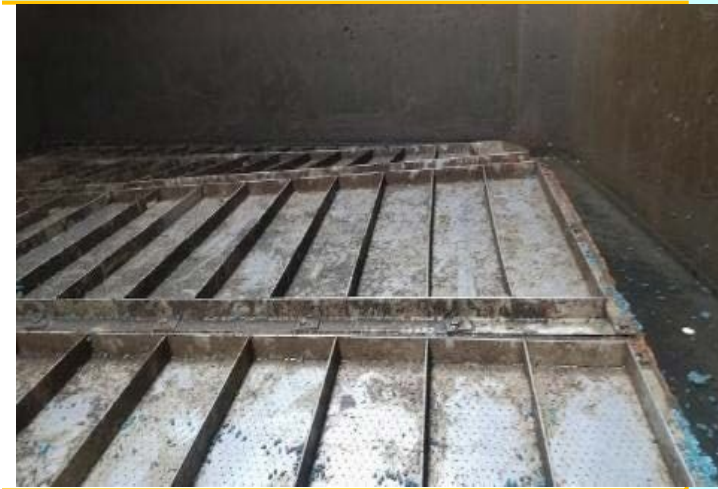
Lifting of steel screen
