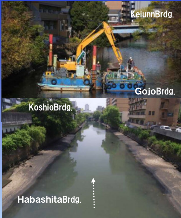
State of middle stream moving on seawall construction (Including sludge dredged)
