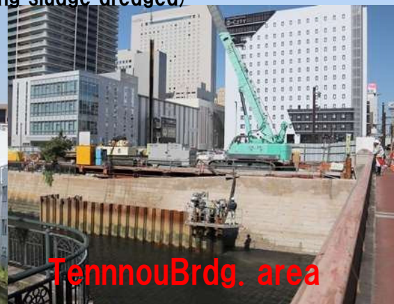
State of middle stream moving on seawall construction (Including sludge dredged)
