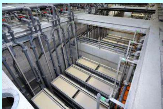
Flat membrane unit aerobic tank
