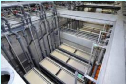
Flat membrane unit aerobic tank (400sheets \times 12units)
