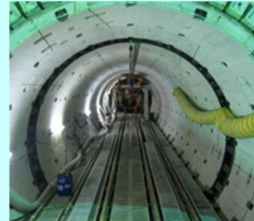
Under construction since 2008 (14,000m 3 )
