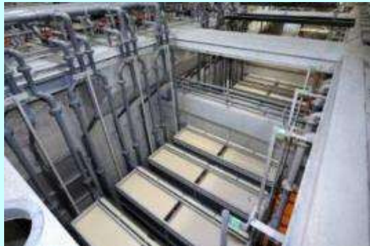
Flat membrane unit aerobic tank (400sheets × 12units)
