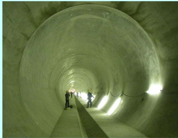
Horikawa Ugan Rainwater Reservoir for pollution control
