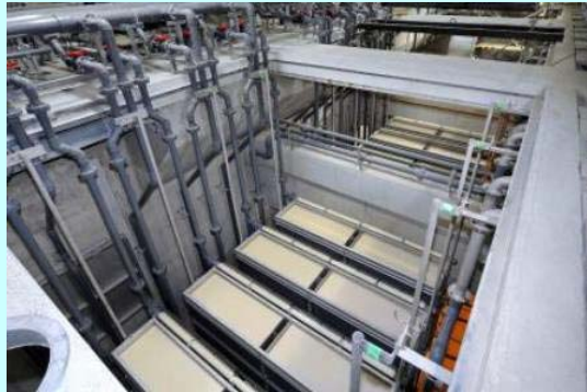
Flat membrane unit aerobic tank (400sheets × 12units)
