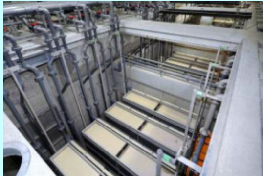
Flat membrane unit aerobic tank (400sheets × 12units)
