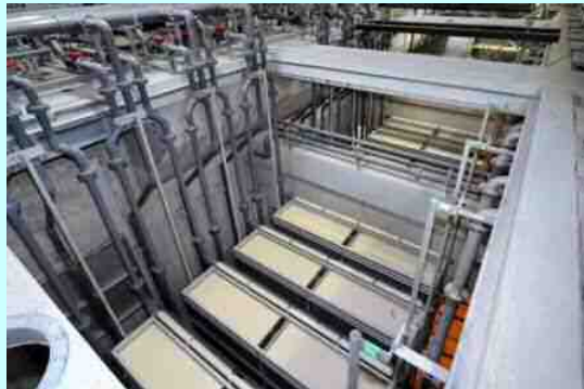
Flat membrane unit aerobic tank (400sheets × 12units)
