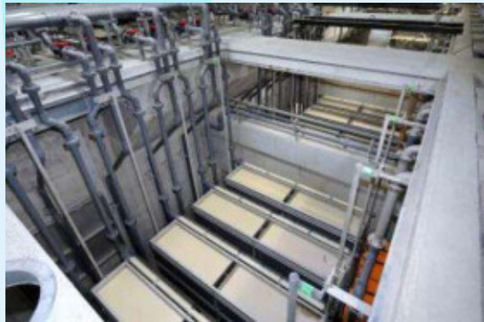
Flat membrane unit in aerobic tank
