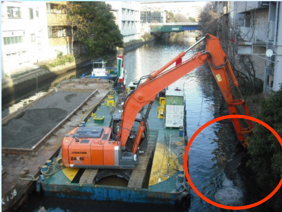
Machines set on a float constructed the experiment site.
