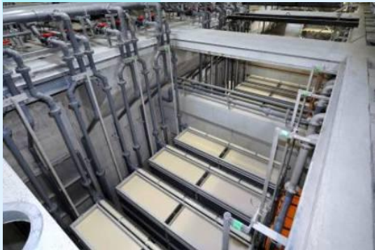
Flat membrane unit in the aerobic tank (400 sheets × 12 units)
