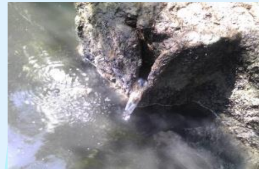
Becoming hollow at sheet pile damaged
